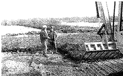
Plate 6.10 A horizon only being placed on a heathland translocation
