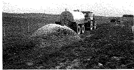
Plate 6.30 Watering replaced heather turves after a pipeline installation at Lazonby, Cumbria
