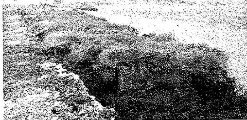
Plate 6.9 1 m-deep turves used for blanket bog translocation
