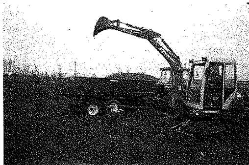
Plate 2.4 Stripping woodland topsoil
